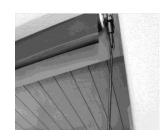
Using provided hand brace, lower shade down slightly and put bottom rail back into pocket of fabric.
